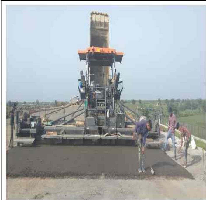
CH 315+300 DLC laying work in progress
