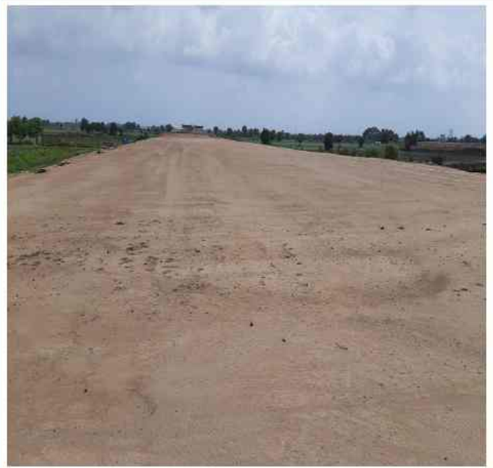
CH 292+000 TO 292+000 SG top work in progress BHS
