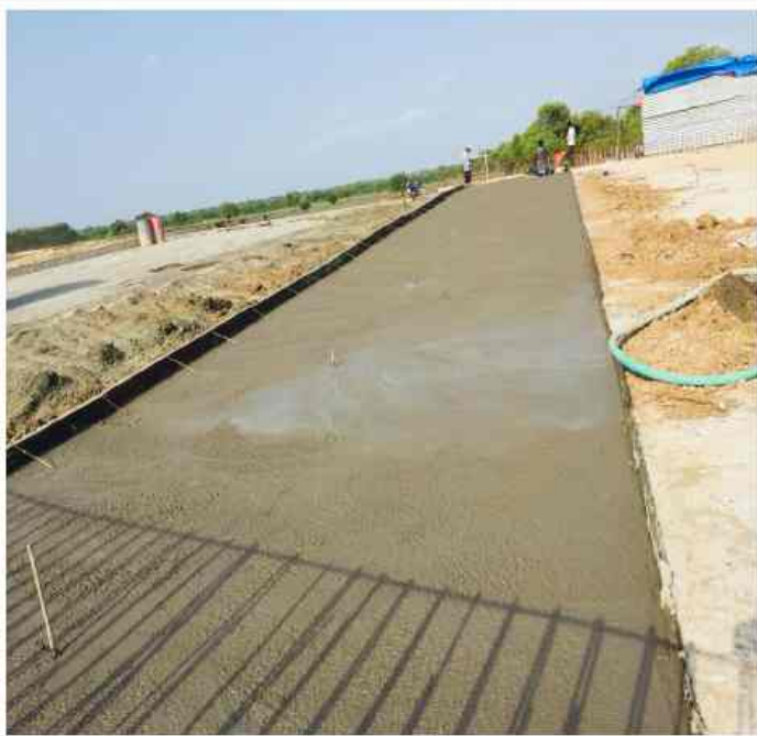
CH 312+695 VUP A2 side Approach slab PCC work in complete LHS
