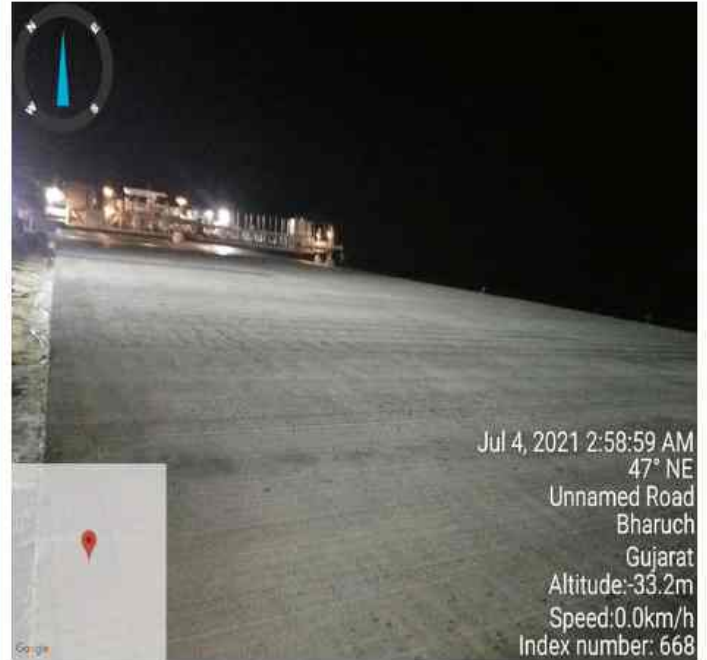
CH 312+420 PQC texturing and curing compound Spraying work in progress
